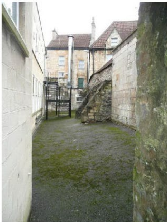
View 1- 4m high retaining wall on rear boundary to the Vintners ( see SK/120 )
